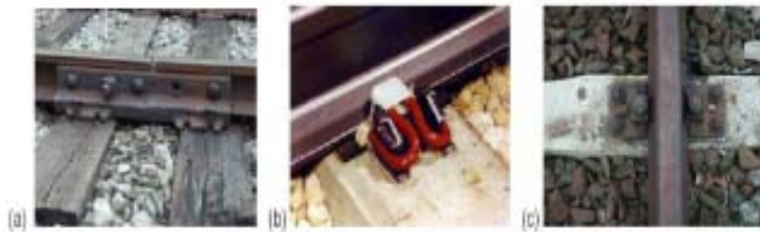
Figure 3 – Common methods of joining and fixing track: (a) mechanically fastened, (b) continuously welded and fixed with clip fastenings, and (c) continuously welded and fixed with AS1 track plates.
