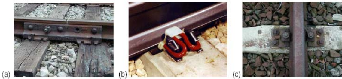
Figure 4.10 – Common methods of joining and fixing track: (a) mechanically fastened, (b) continuously welded and fixed with clip fastenings, and (c) continuously welded and fixed with AS1 track plates.
